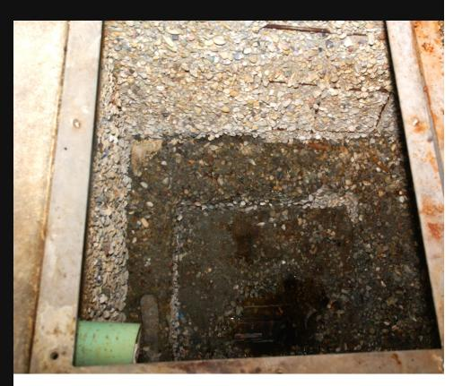
The pictures pretty much tell the story here, this sump pit was dried, cleaned, scarified and trowelled with a high strength repair mortar. The mortar was allowed to dry for four hours, lightly diamond grinded and trowelled with Tnemec 243 a vertical grade Urethane Cement. The entire project was completed in one day and put back into service the following morning.
