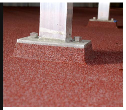
A Central Coast winemaker near Paso Robles California wanted a durable floor that was aesthetically pleasing. Ucrete HPQ was recommended and subsequently installed, it was selected because the color quartz finish provided slip resistance and was ascetically pleasing. The floor was 1/4" thick with a Polyure-thane Cement base that is incredibly durable. A 6" Integral cove base was installed in many of the rooms as well as a 45 degree radius at the column bases.
